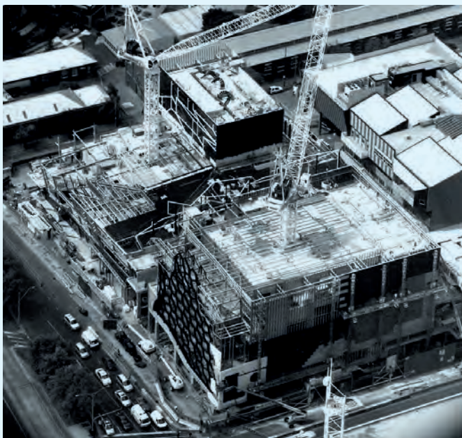
Melbourne Recital Centre in construction, 2008
